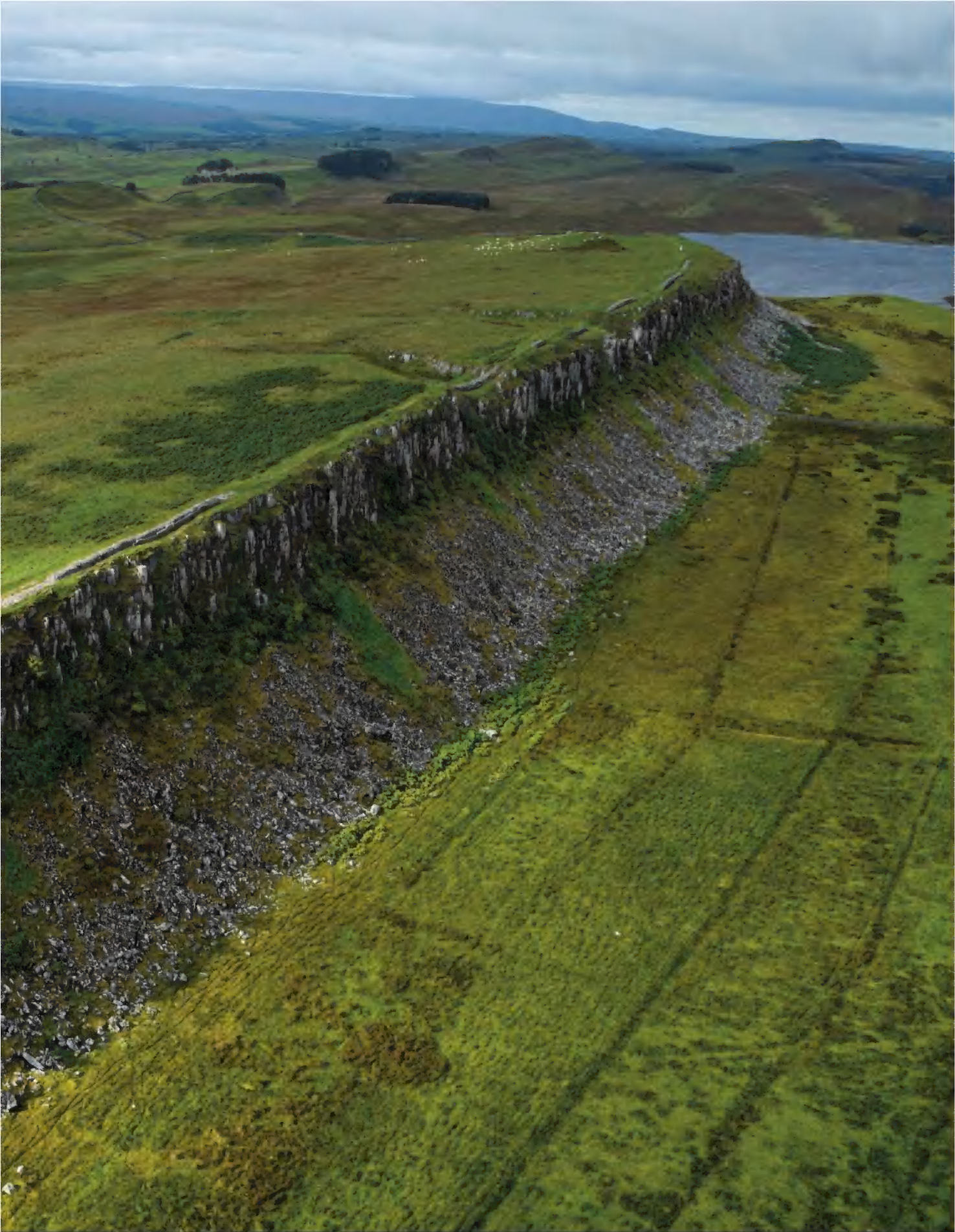
HADRIAN'S WALL, ENGLAND Barbarians would have stared up at this section, which runs along a cliff near the northern town of Once Brewed. In its heyday, the wall was 14 feet high and stretched 73 miles, from coast to coast. A deep ditch reinforced parts of it. Today a walking trail runs alongside it.
